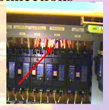
Hot Spot Temperature.....459F Reference Temperature.....101F Temperature Difference....358F
