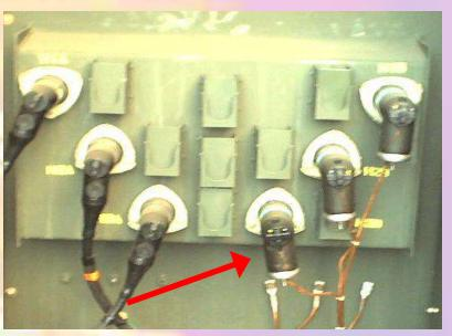
Hot Spot Temperature....92F Temperature Difference..32F Ambient Temperature....45F
