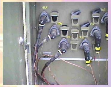
Hot Spot Temperature....159F Reference Temperature....98F Temperature Difference...61F Ambient Temperature....71F
